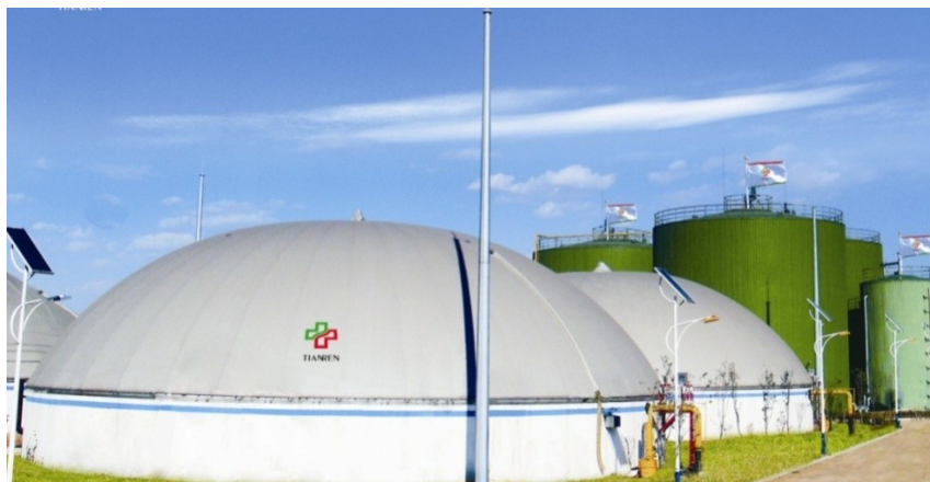
Figure 14 • Vehicle fuel biogas plant producing (Anyang, Henan Province)
