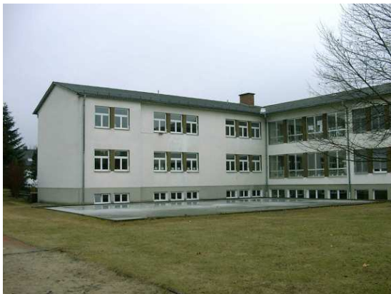
Figure 31: Old public building with forfeiting-EPC – picture of the facade
