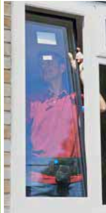
Full window replacement
