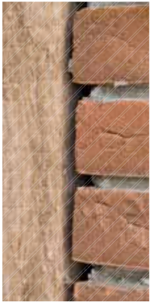
Cavity wall insulation
