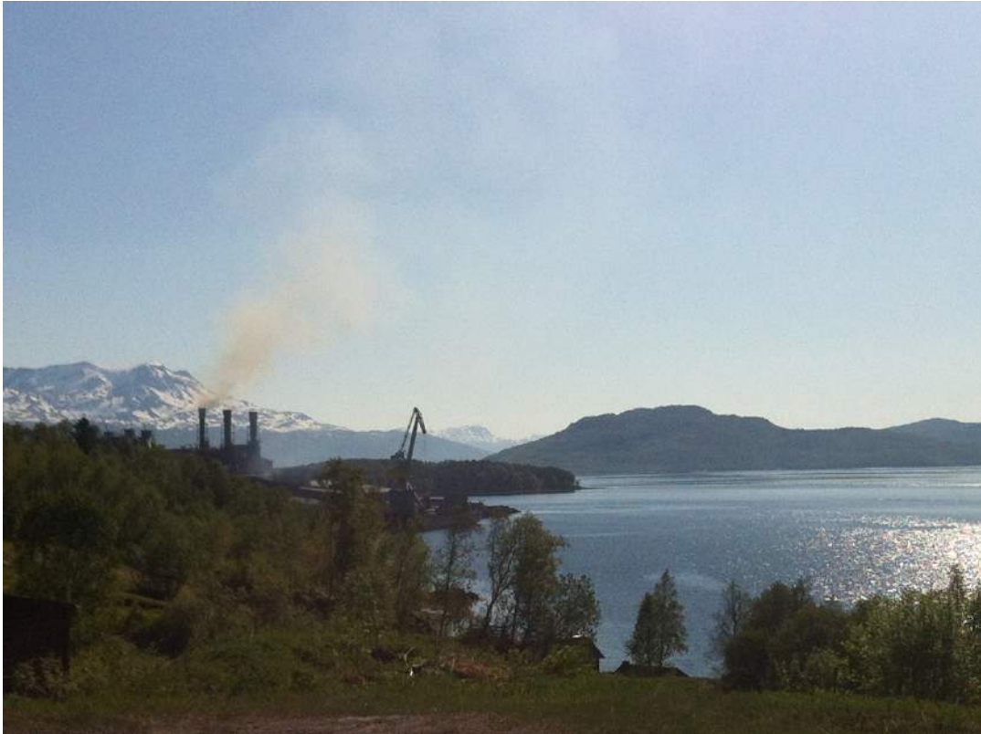
The beautiful setting of Finnfjord, the world's most energy efficient ferrosilicon plant
