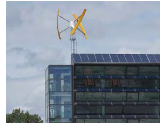
SWT on the ENERGYbase
