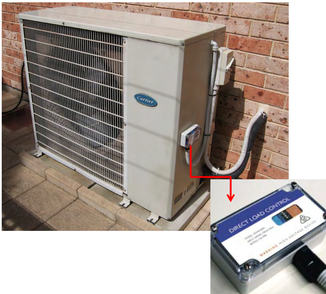
Figure 4. Saab Systems “Peak Breaker” Direct Load Control Device Used in the ETSA Utilities Air Conditioner DLC Phase II Project
