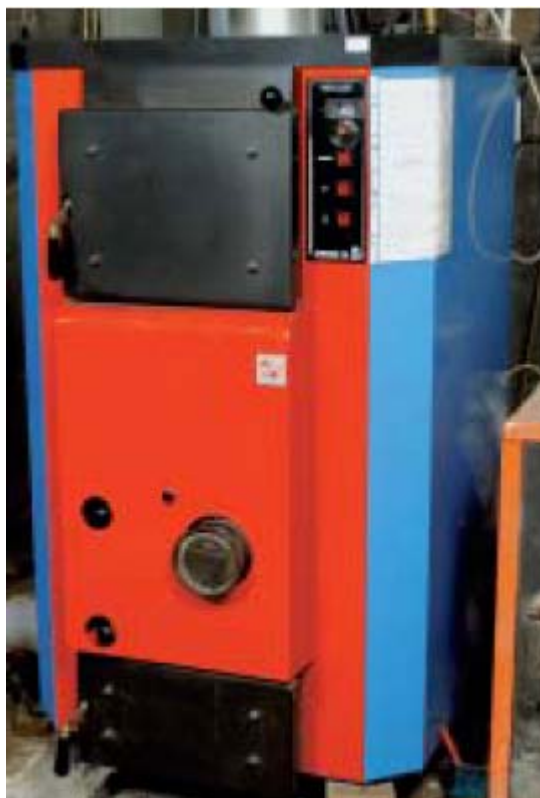
Figure IP06/4. Wood-fired Boiler
