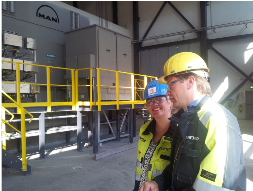
Figure 1. IEA-DSM Operating Agent Sea Rotmann being shown around the heat recovery plant by Finnjord CEO Geir-Henning Wintervoll. Photo: Henrik Karlstrøm
