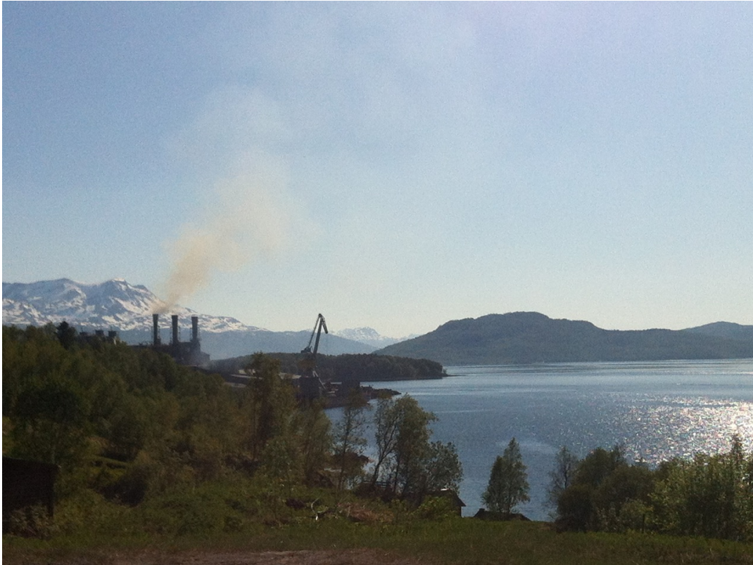
The beautiful setting of Finnfjord, the world's most energy efficient ferrosilicon plant
