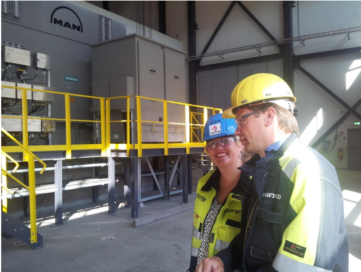
IEA-DSM Operating Agent Sea Rotmann being shown around the heat recovery plant by Finnfjord CEO Geir-Henning Wintervoll. Photo: Henrik Karlstrøm
